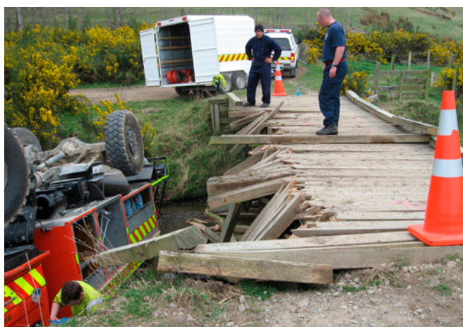
Figure 3.2 Check bridge for load rating
