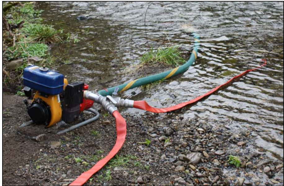
Figure 4.5 – Bypass hose in operation in cleared area
