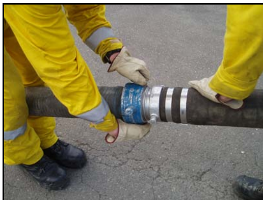
Figure 4.5 – Hand tighten suction hose couplings
