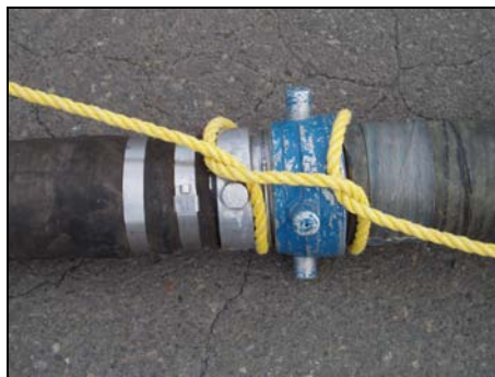
Figure 4.8– Supporting the suction hose
